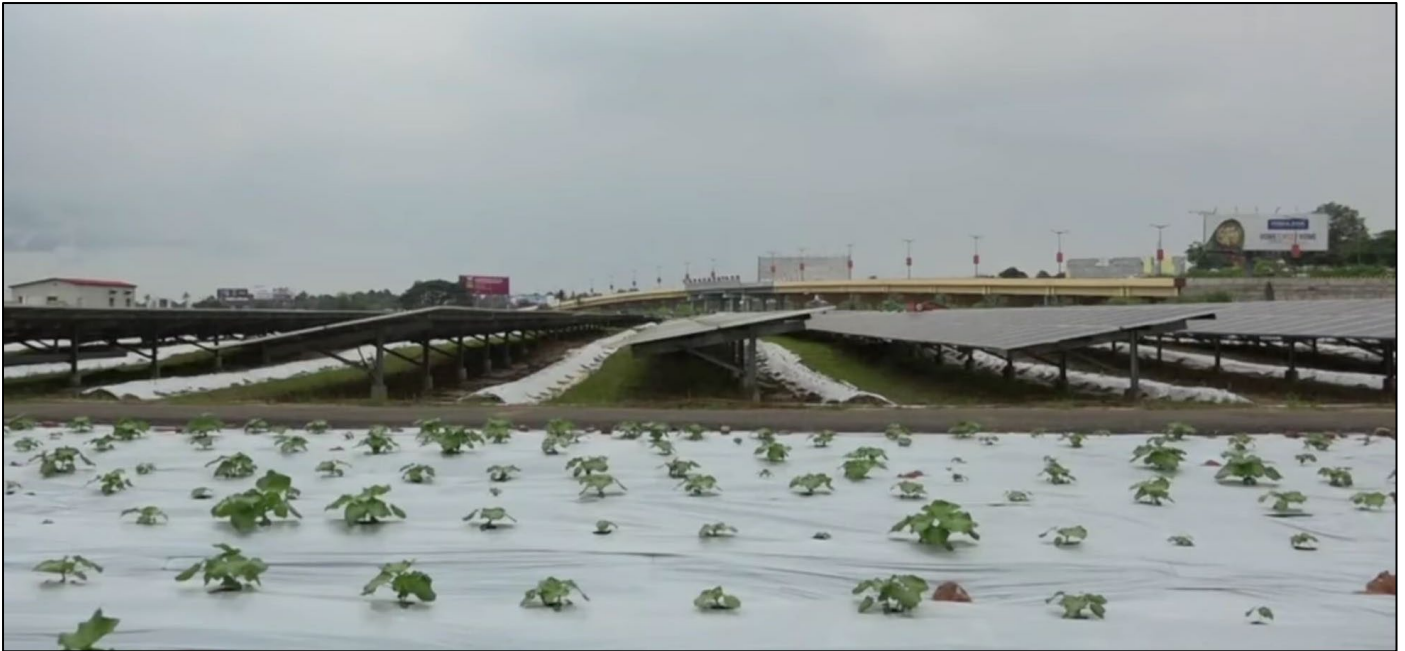
Figure 18: Agrivoltaic plant at Cochin Airport (Credit: CIAL)
