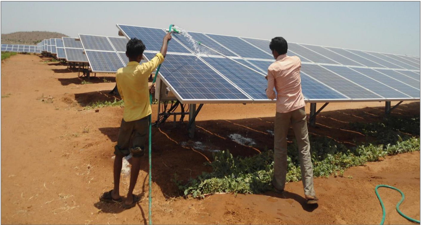
Figure 10: Cleaning and irrigation at Abellon Energy plant (Credit: Abellon Energy)
