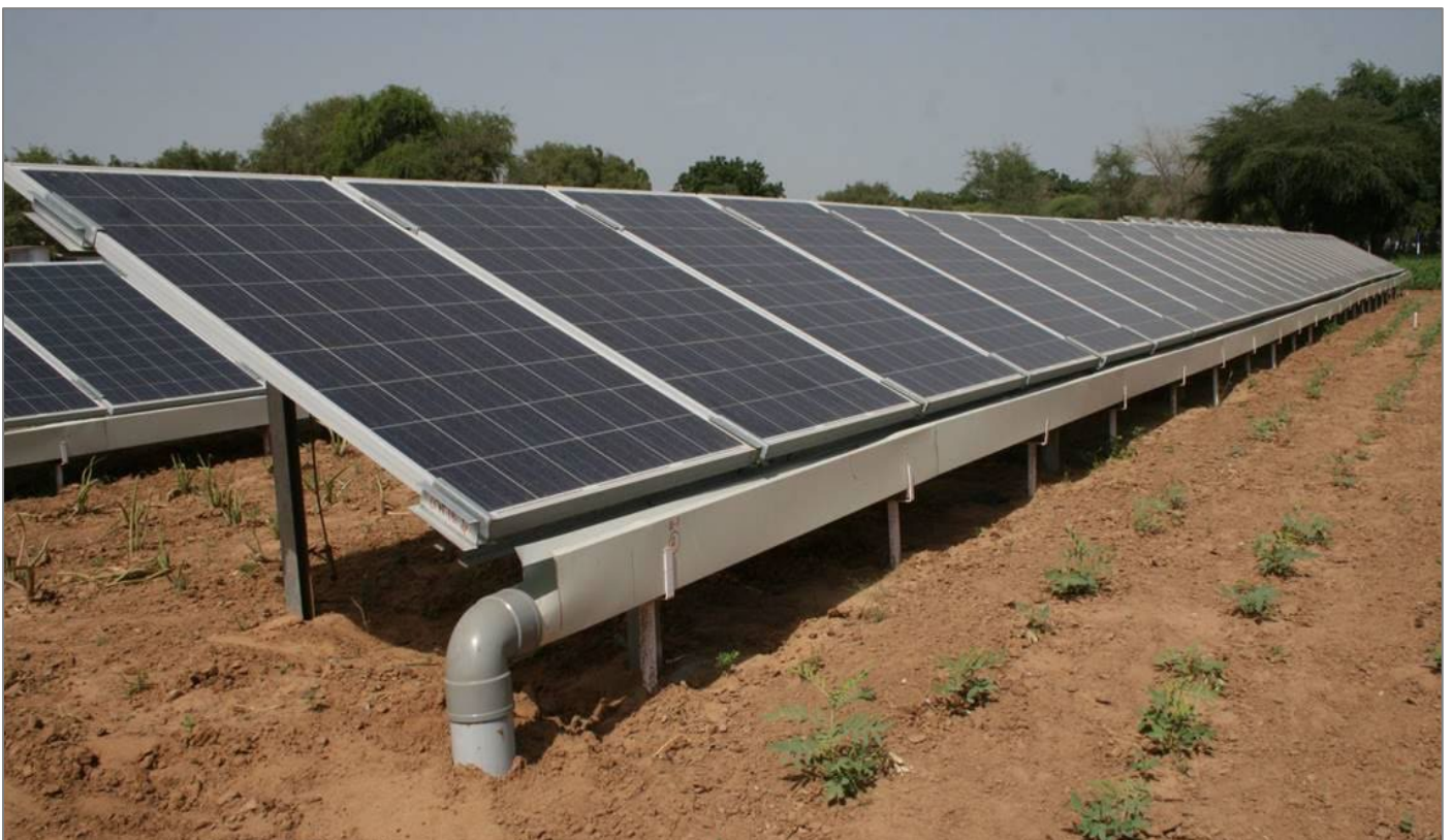
Figure 3: Agrivoltaic system with rain gutter at CAZRI (Credit: CAZRI)
