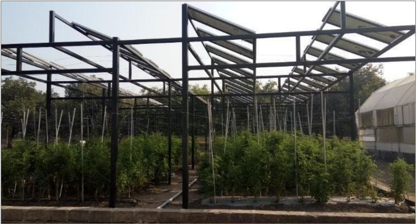
Figure 7: Junagadh agrivoltaic system (Credit: Prof. P.M. Chauhan, JAU)
