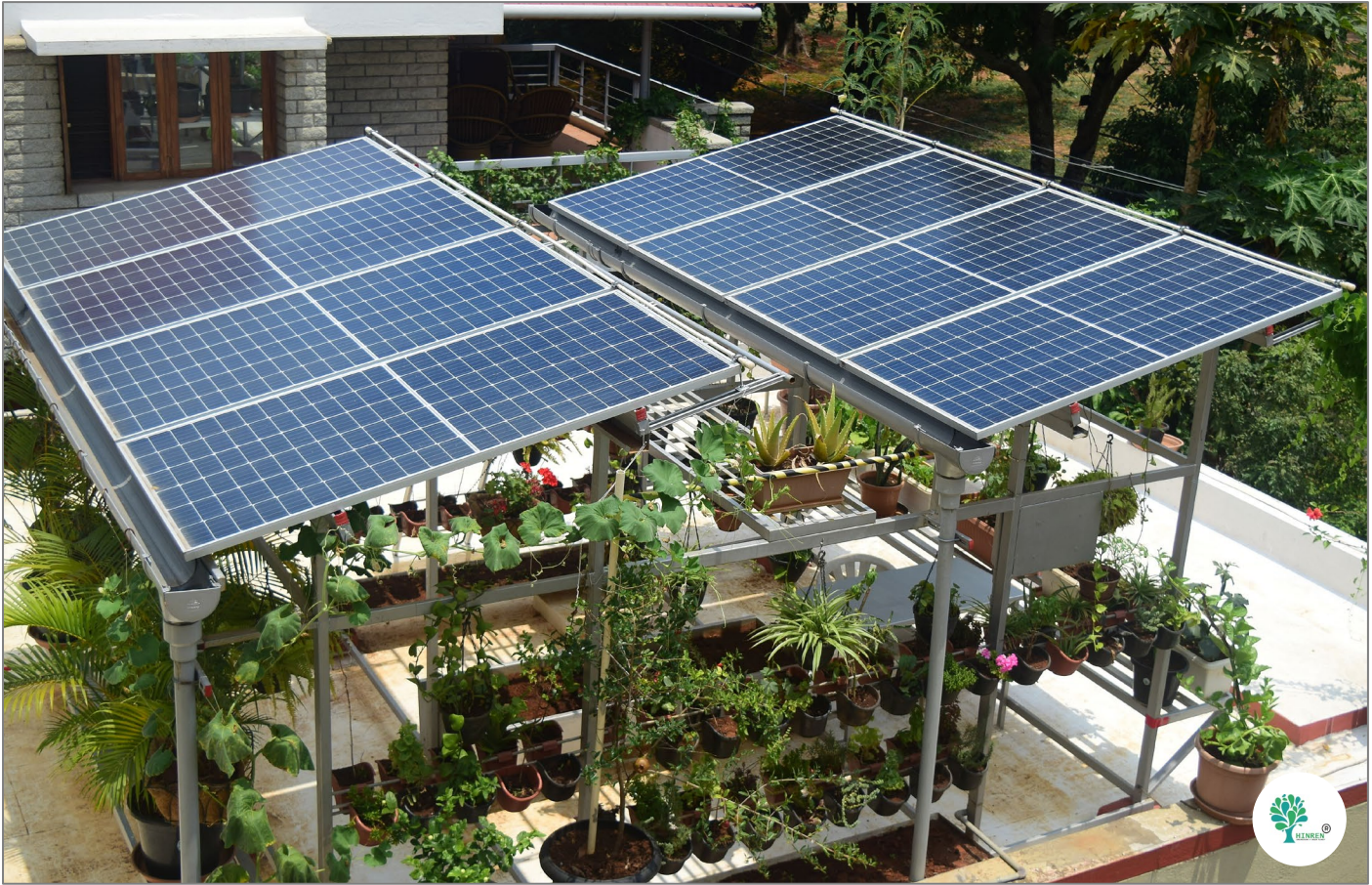
Figure 22: Hinren Agri-PV rooftop system (Credit: Hinren Engineering Pvt. Ltd.)
