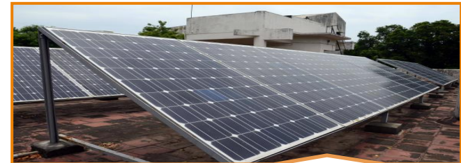
Rooftop SPV installation at Municipal School
