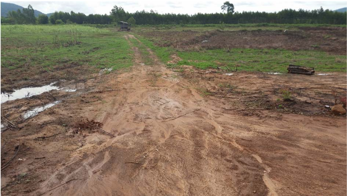
Figure 22: High amount of eroded soils
