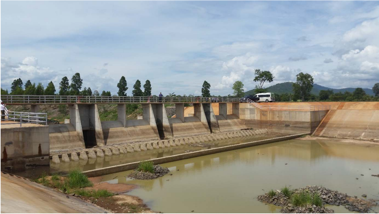
Figure 34: Big weir with shaped backwater area
