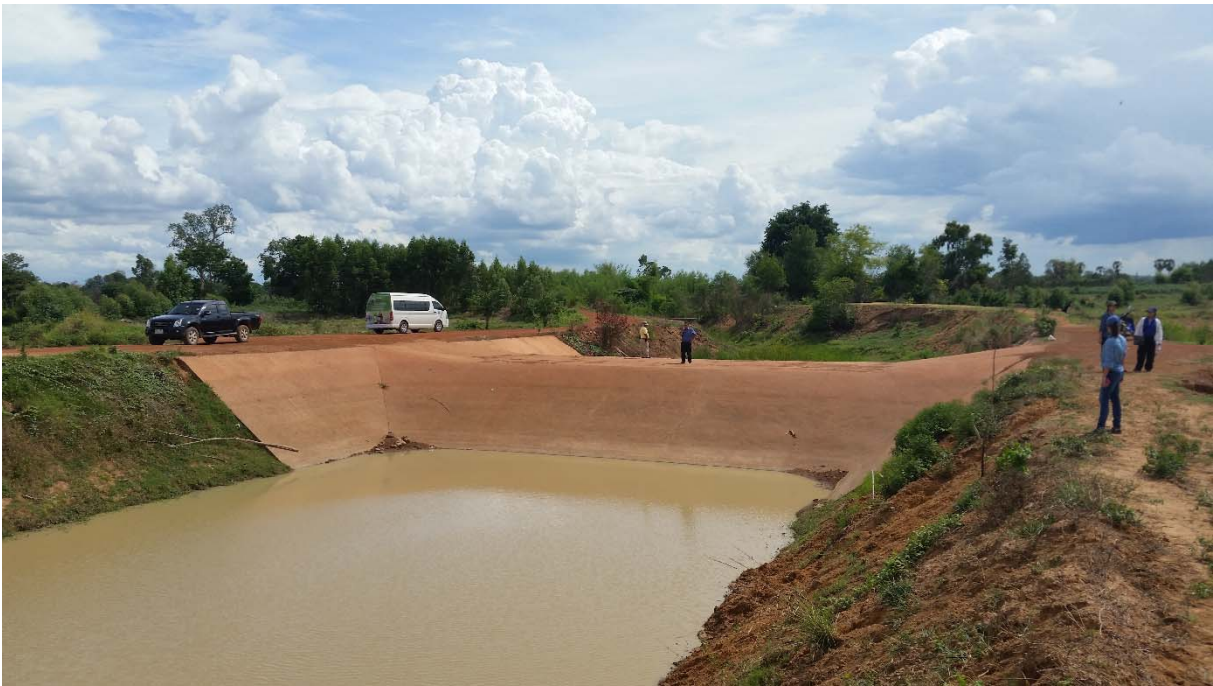
Figure 33: Concrete weirs (without gates)
