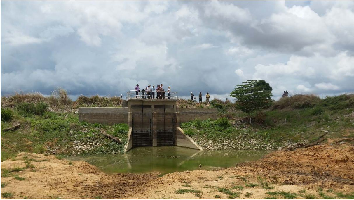
Figure 32: Concrete weir (with gates)
