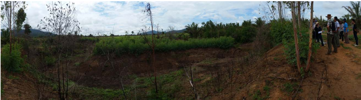
Figure 39: Area at the dam site
