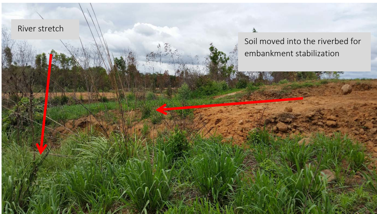
Figure 27: Stabilization of river embankment with fertile soil
