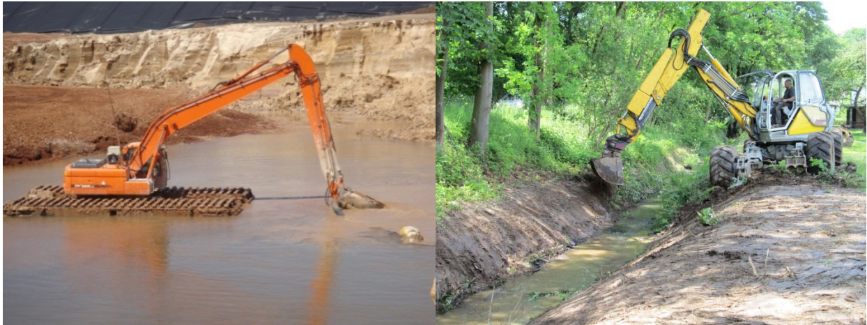
Figure 5-12: Example of reservoir dredging (left) (Source: http://belldredgingpumps.com/amphibious-excavator/ ) and river dredging (right) (Source: Zumbroich Consulting).
