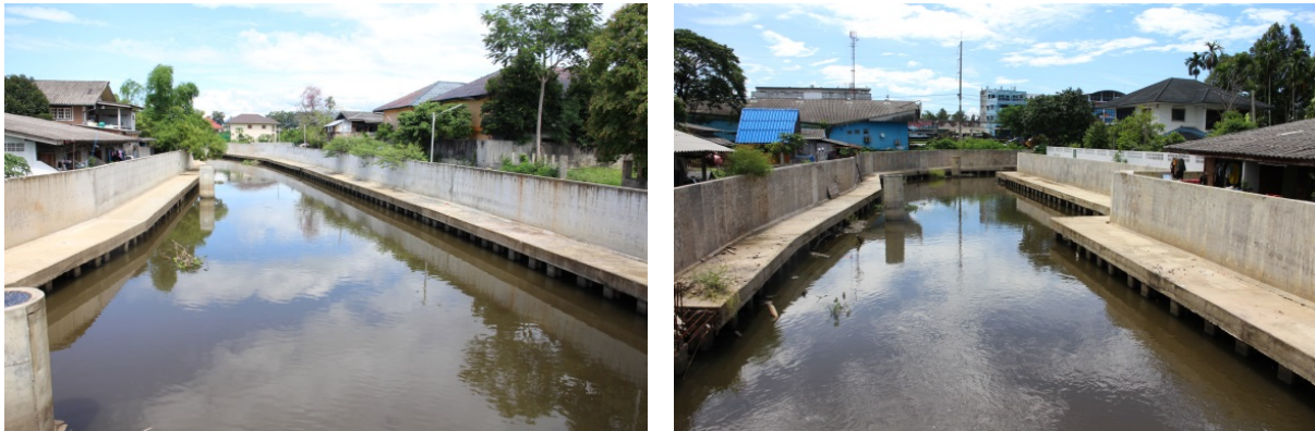
Figure 6-5. Flood protection walls constructed downstream in Nakhon Si Thammarat
