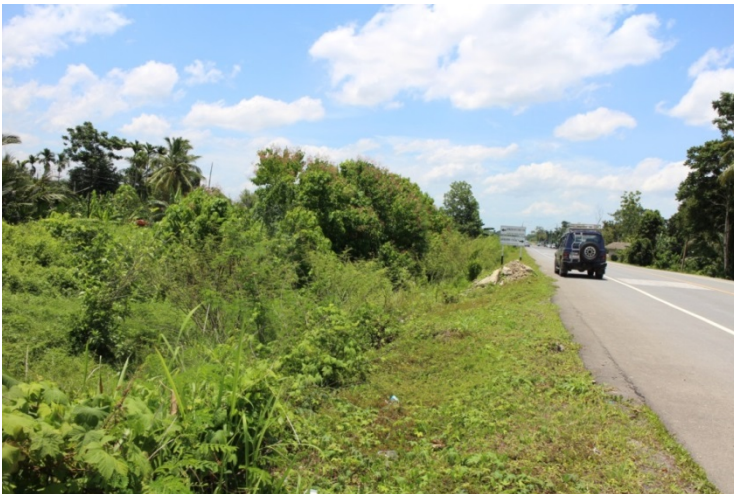
Figure 6-8. Space between the railway and the road which could be inundated during high streamflow periods and create a wetland
