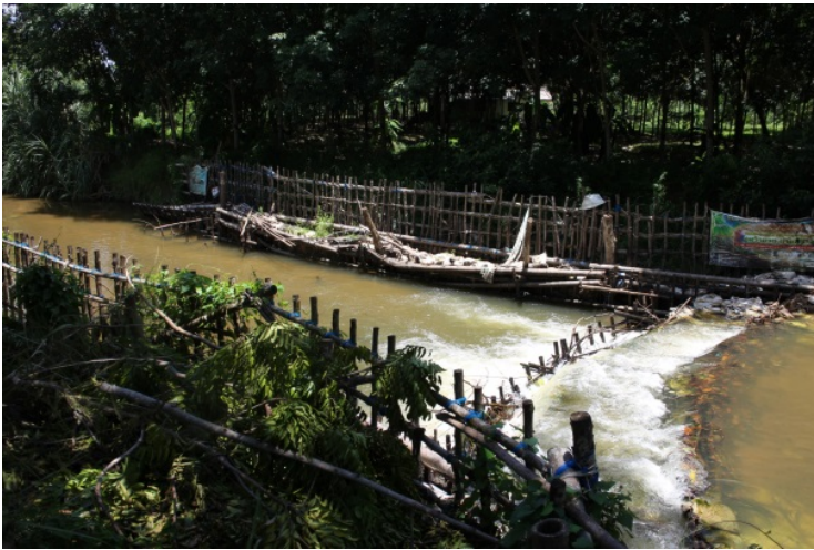
Figure 6-7. Example of a living weir with river bank stabilisation in the Tha Di river
