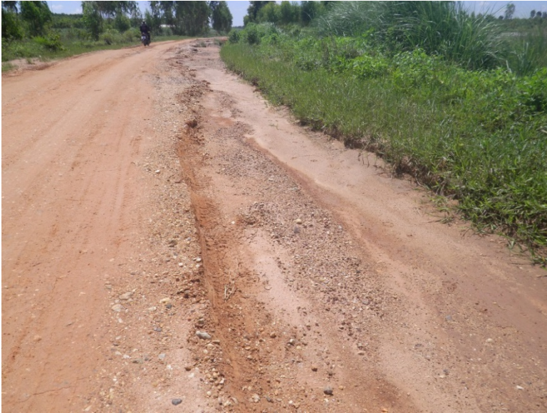
Figure 5-6: Erosion of fine sediments along unpaved road in the upper part of the Huai Sai Bat Basin (Photo: G. Meier, 2015).
