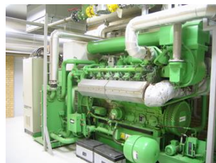
Figure 1. Thermal oil heater and gas engine at a Tapioca mill
