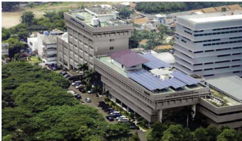
The PV system on the rooftop of Asean Centre for Energy building in Jakarta
