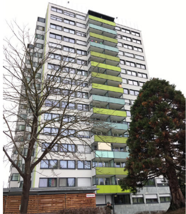
Visit of Buggi 50 – the first retrofitted passive tall building in Europe 访问Buggi 50 – 欧洲第一座改建的高层被动式建筑
