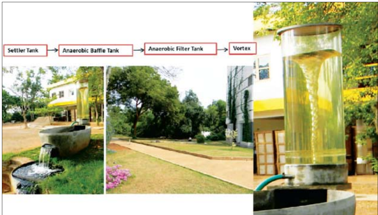
Image no. 3-27: Decentralized treatment system with schauberger vortices
