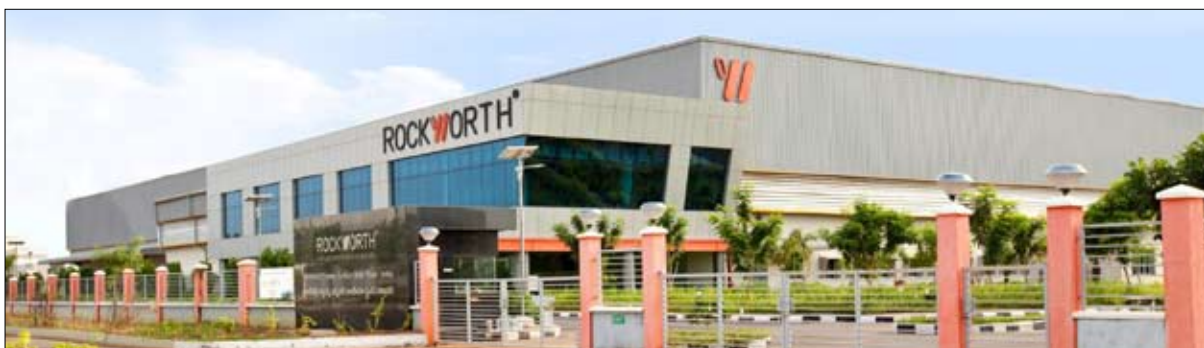
Image no. 3-16: Examples of green factory buildings at Sri City, Tada, Andhra Pradesh
