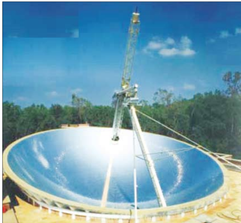
Image no.3-23: Solar bowl at the solar kitchen- Auroville's community kitchen [Source: The Power of Human Unity. (n. d.). Solar Bowl at the Solar Kitchen - Auroville's community kitchen . Retrieved from http://www.aurore.in/the%20power%20of%20human%20unity%20june_2004.pdf ]
