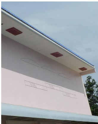
Installation of roof vent in the eaves
