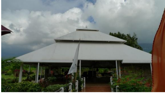
Rainwater harvesting (the rainwater that falls on the tent is collected in an underground tank and used for irrigation purposes)
