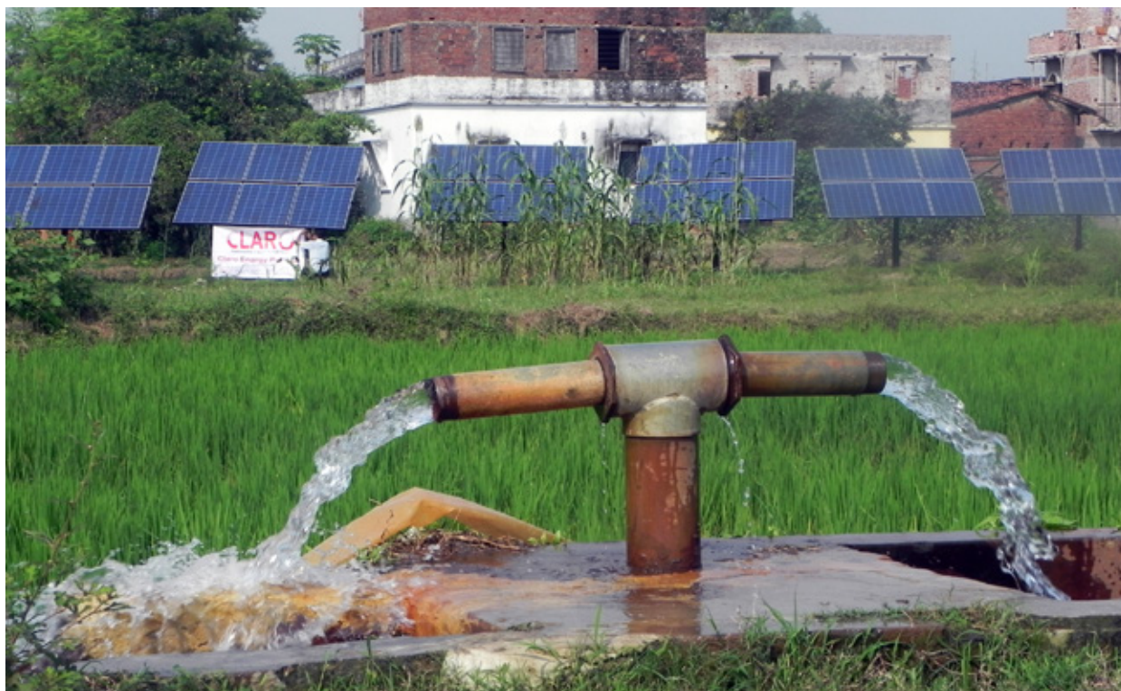
Solar pump with tracking system by Claro Energy Pvt Ltd. Picture Courtesy: Claro Energy Pvt Ltd.
