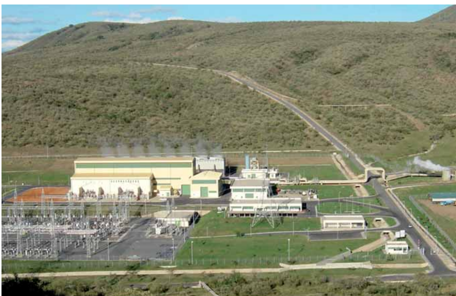
The largest geothermal power station in Africa: Olkaria II in Kenya.
